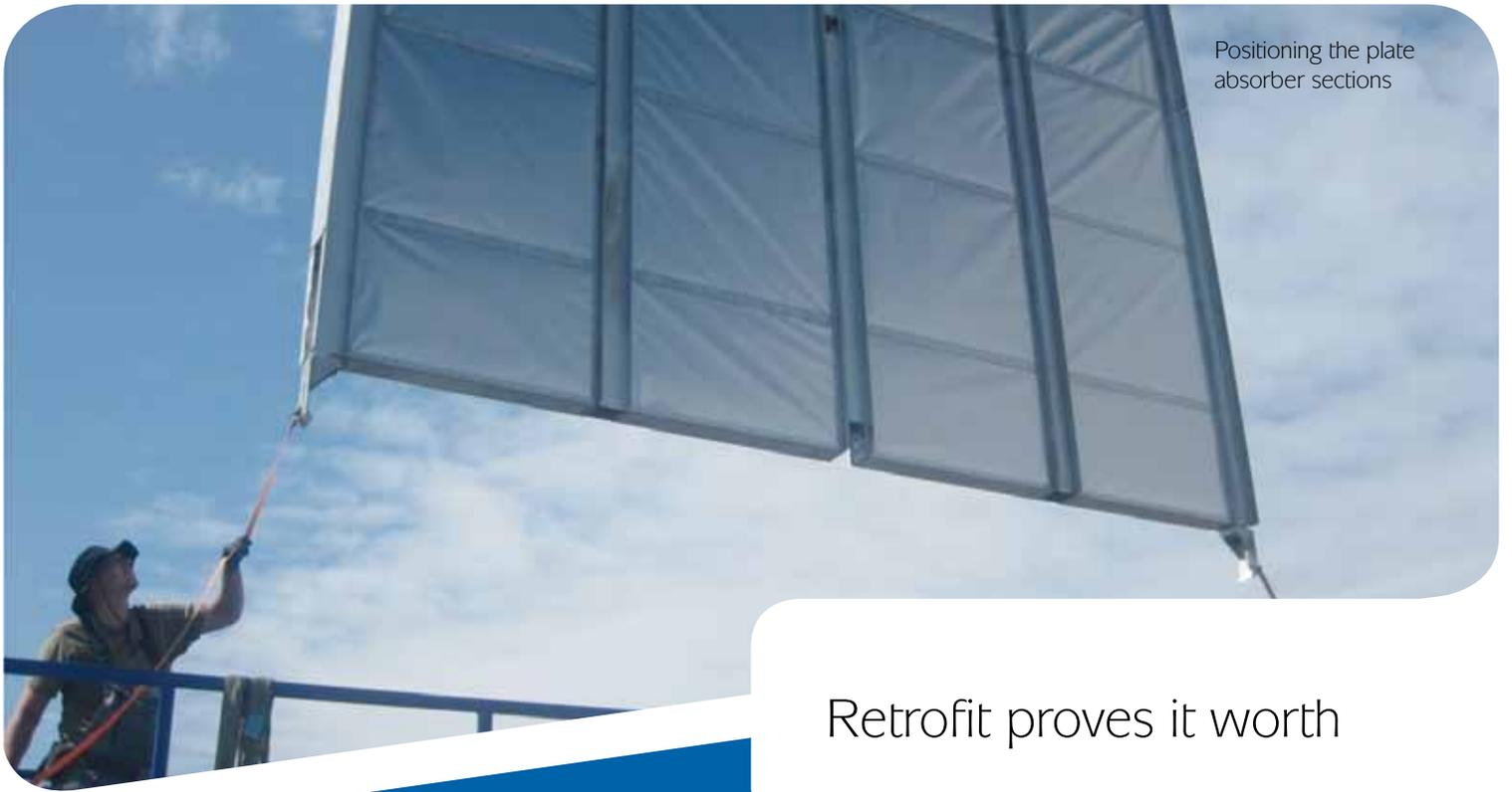
Positioning the plate absorber sections
