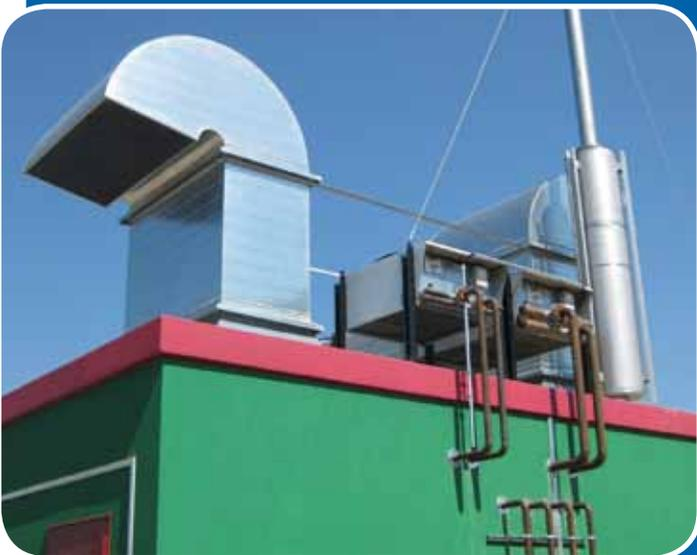
Typical exhaust gas silencer installation for a biogas plant. The main priority here is the elimination of low frequencies (engine ignition frequency)
